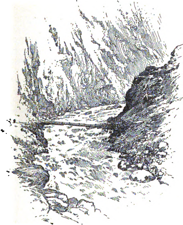
SHAITAN NARA, OR THE DEVIL'S BRIDGE. CANTILEVER BRIDGE OVER THE ASTOR RIVER.
